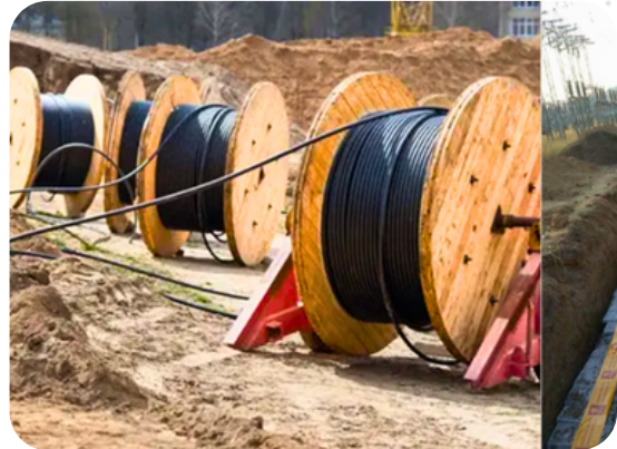
Underground Cable & OFC Works
